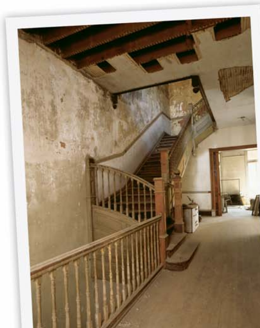
Left: All of the stairway parts were removed, stripped, refinished and reinstalled throughout the hotel.
