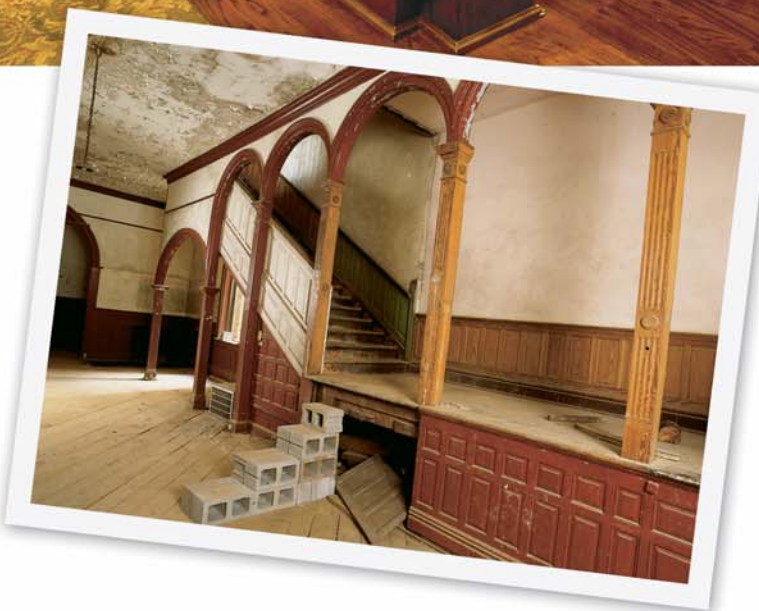
Left: All of the stairway parts were removed, stripped, refinished and reinstalled throughout the hotel.
